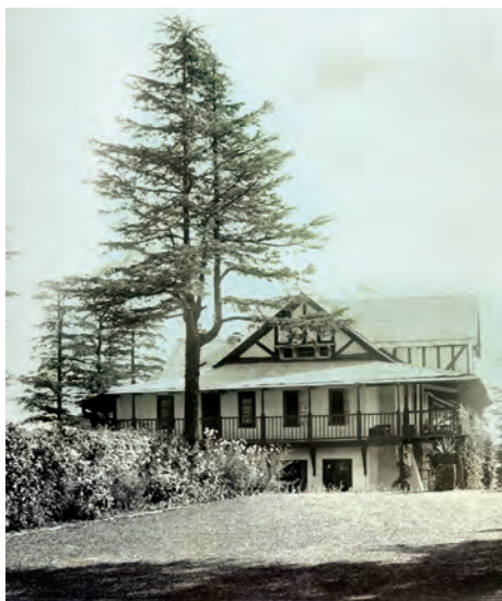
Fig. 12.12 A typical colonial house in Simla, an early-twentieth-century photograph
